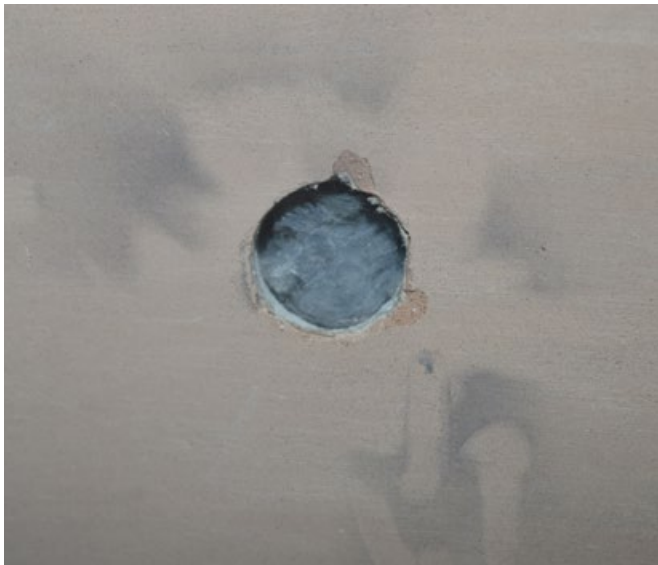
Figure 9: Spacefill in situ, after it had been blown into the cavity.
