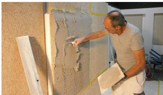
Figure 11: Application test of the insulating mortar ISOCAL
