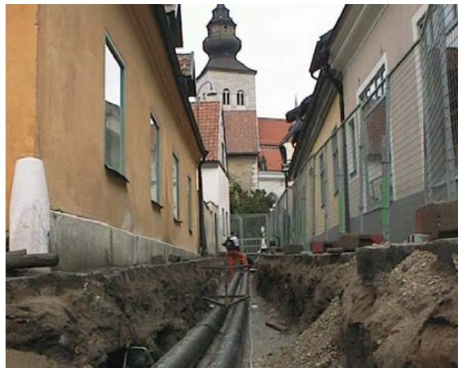
Figure 45: Installation of a district heating system below the streets of Visby’s historic city centre, a World Heritage Site (Image © GEAB)
