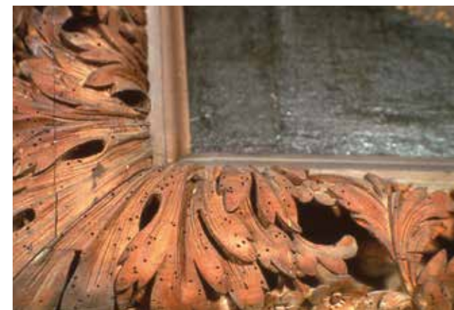
Woodworm damage (National Trust Images)
