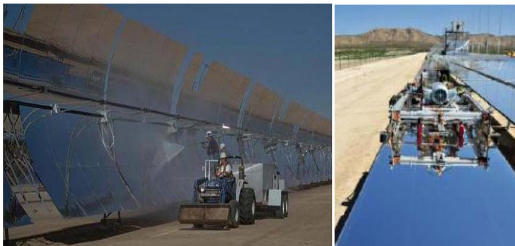
Figure 32 left: Conventional cleaning methods (Cohen, 1999), right: water-efficient cleaning using a cleaning robot of Fresnel collector by Novatec Biosol (Novatec, 2010)
