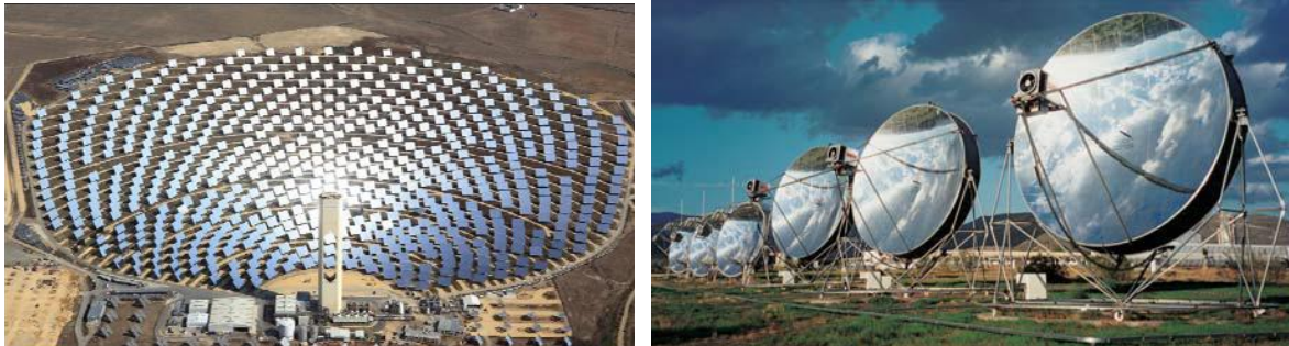
Figure 3 Point-focusing systems: Left: Solar Tower plant PS10, 11 MW el in Seville, Spain; 624 so-called heliostats, 120 m 2 each, focus the sunlight onto a receiver on top of a 100 m high tower (Abgengoa, 2010). Right: Dish Stirling prototype plants of 10 kW el each in Almería, Spain; diameter 8.5m (DLR, 2010)
