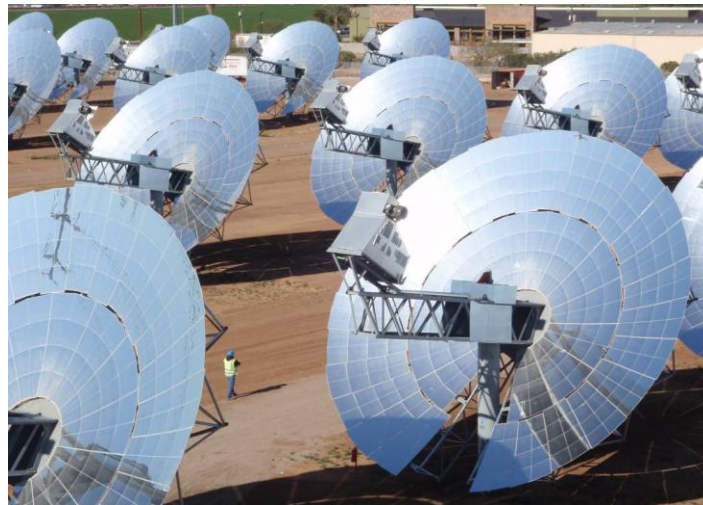
Figure 9 Maricopa Dish Stirling Farm in Arizona, the park has a rated power of 1.5 MWel consisting of 60 Dish-Stirling units
